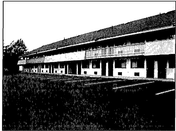
Block 1310 Lot 12.01 looking N/W
