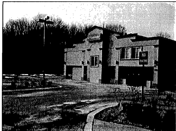
Block 1310 Lot 10.01 looking S/W
